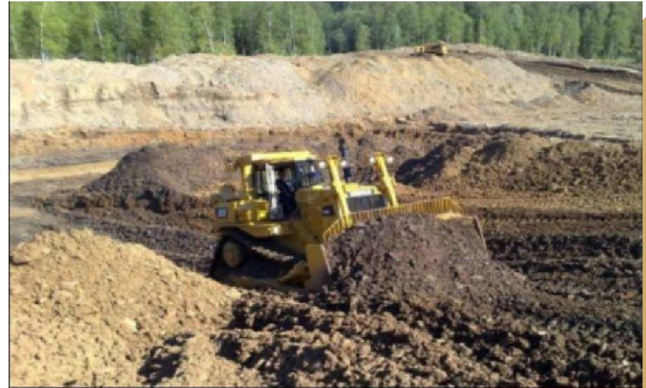
Gold-bearing sand being moved to the crushing facility
